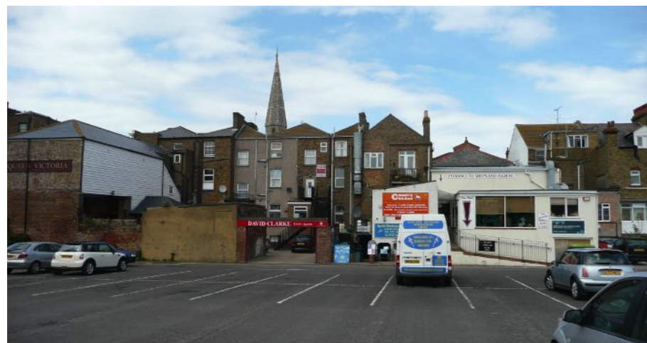
View of existing service access points in William Street car park, to rear of existing High Street properties
