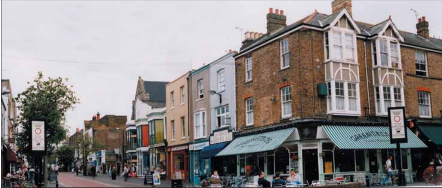
Mortimer Street looking east from the junction with William Street. A range of building, and building alteration, dates is visible. The corner building is Regency in origin, with Victorian bay windows and a (probably) early 20th century shop front. The town's Congregational Chapel occupies the street front gap in the middle distance.
