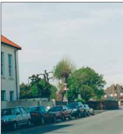
View from the Roman Catholic primary school, west along Avenue Road and out of the conservation area.
