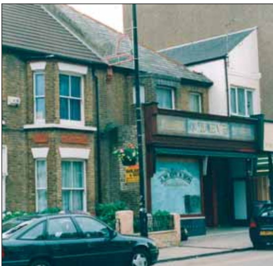
A precursor to a world of two storey semis after the First War. Paired bay windows with doors at each side. Half of this example has lost its front garden to a later shop, 1875-80. High Street close to Station Road. junction.
