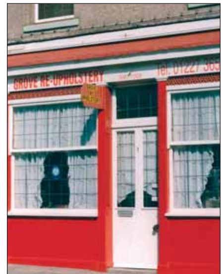
Simple shop front in New Street with Victorian tall and wide sash windows, small signboard above and, on top of this, a large, added, blind box. The small panes are the modern stuck-on sort not historically related to the original design of the sashes.
