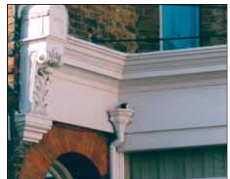
Top left: Nicely carved acanthus leaf style console brackets on a single storey Victorian shop extension to a house, New Street.
