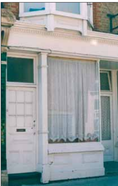
Pilaster and cornice etc 'enclose' from left to right, door to flats above, shop window and shop entrance, East Street.
