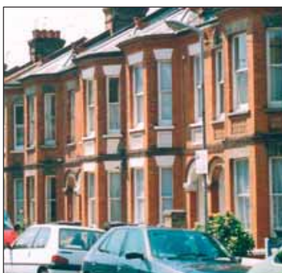
Finely detailed terrace with full height two storey shallow hipped-roofed canted-sided bay windows. Late 19th/early 20th century.
