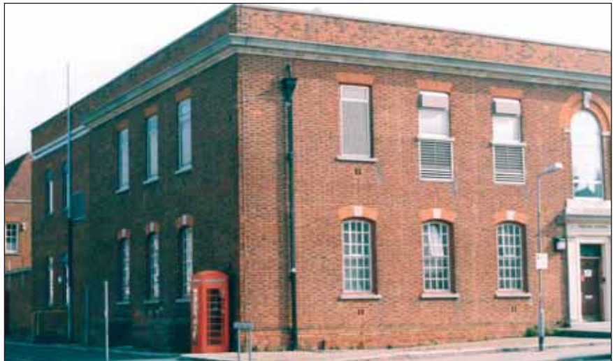
Second purpose built Post Office and Telephone Exchange (nearest camera) Cavendish Road.
