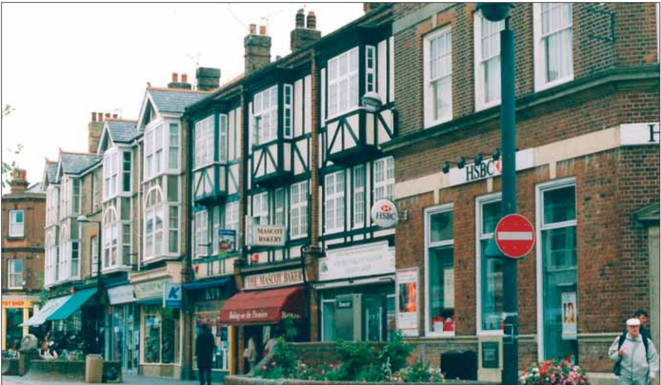
William Street looking towards Mortimer St. Bays at second floor level.
