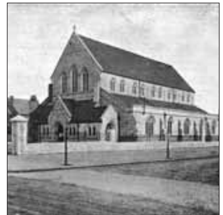
St John's Church in Brunswick Square. Subsequently demolished.
