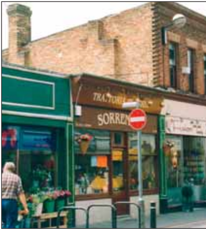
Single storey shops, Mortimer Street. Note toothed brickwork to first floor facade.
