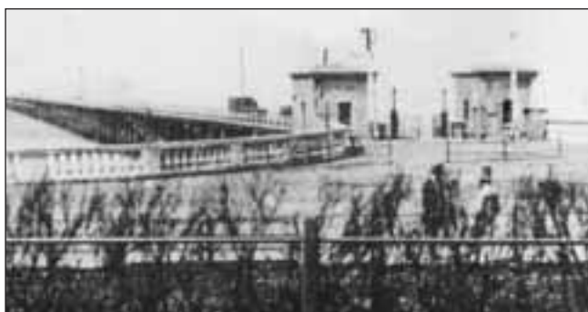
The first pier.
