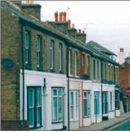
Above: Tiny single storey bay windows on later 19th century artisan housing. Market Street.
