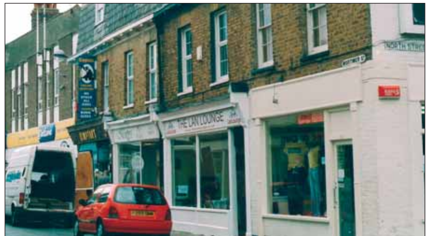
Shop fronts inserted into early 19th century houses –“front” doors open into shops only, Mortimer Street.
