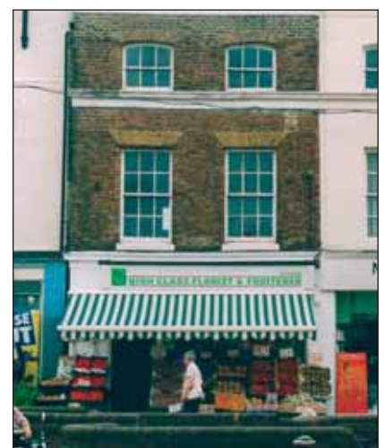
Pair of houses, Mortimer Street. Later shop fronts.
