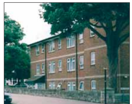
Modern central development within Brunswick Square. Elevation to Station Road.
