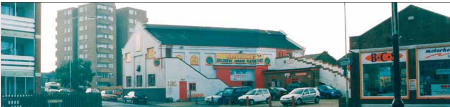
View south across King's Road from corner of 7 storey tower block (left) to former gas works buildings site. 10 storey tower block looms behind, eastward across the main road. Exposed parking arrangements for cars dominate the scene.
