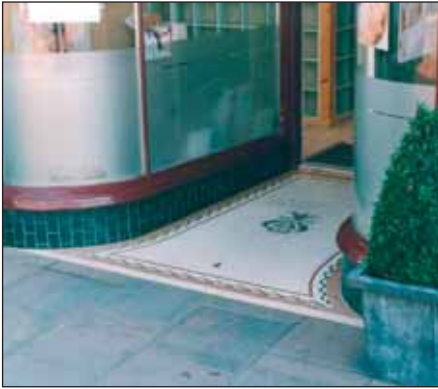
Curved glazed tile stall-riser and tiled in-go. 1920/30s.
