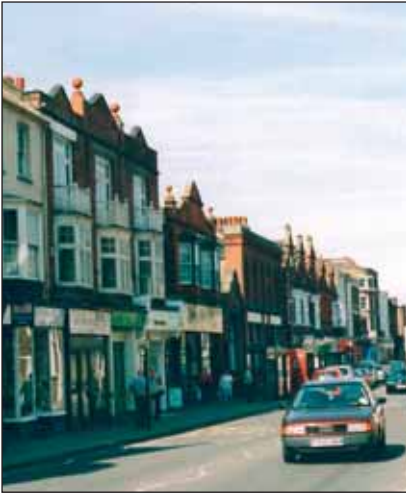
The library - the building with a parapet - had now been built to fill the last gap in the south side of the High Street beyond William Street.
