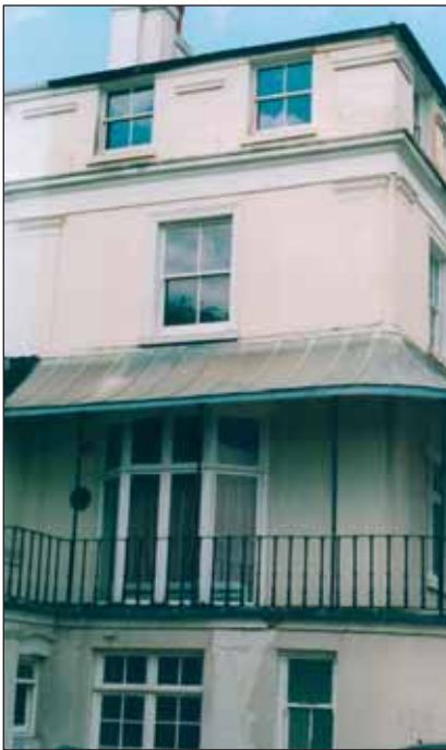
Corner detail of 1835 house group at Oxenden Square/Oxenden Street junction.
