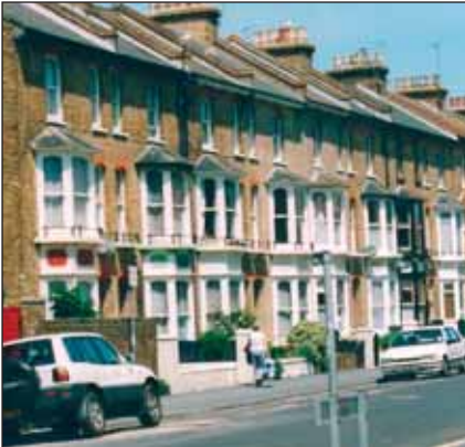
Three storey terrace with two storey bay windows, later 19th century, designed, as are all examples here, to meet the Housing Act criteria. Note the fire break walls. South Road. 1890s.
