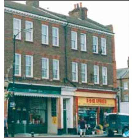
Circa 1900, North Street/High Street junction.
