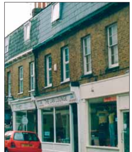
Mortimer Street: original first and second (mansard) floors. Rare cornice gutter. Later shop fronts.
