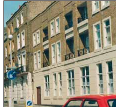
Considered attempt at marrying historic and new housing together, 1990s. 'Chislet Court' former Cinema site on Avenue Road.
