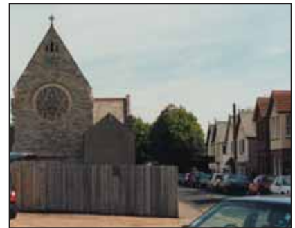
View from end of garage forecourt, York Road, looking north east down Clarence Road. South west end of Catholic Church on left.
