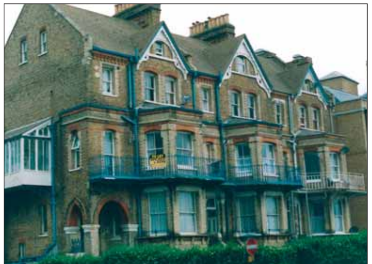
Block of 3. Non-handed plan. Bays to all 3 dwellings. No bay to top floor but gable introduced above notwithstanding. Special corner entrance detail. Iron balcony arrangement at first floor level may be original. Canterbury Road.
