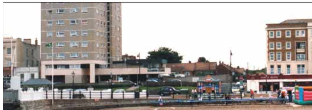
St George's Terrace, the tower block on the Pier Hotel site and the Pier pub, seen from the Pier.
