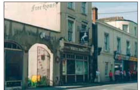
The street front of the White Horse today. This is a 'threatened building', derelict and a potential target for vandals. The two storey elevation to the right masks an earlier arrangement in which the curved corner at second floor came lower down.
