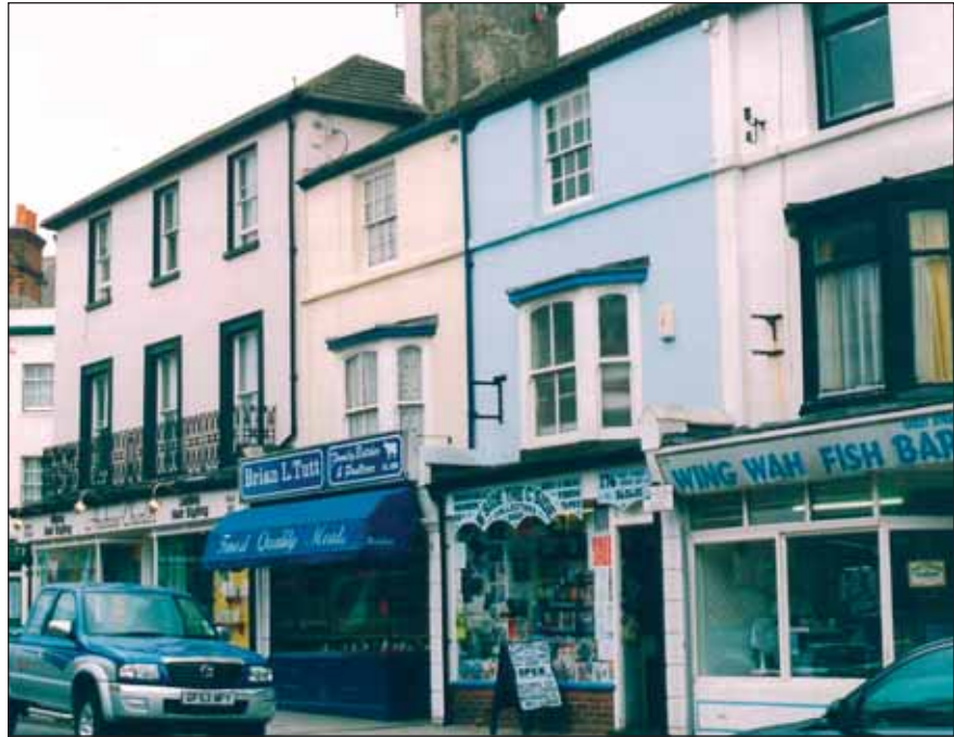
Added-on shop fronts. Left: Four Fathoms pub, High Street. Victorian pierced masonry balcony. Right: Garibaldi Terrace, High Street.
