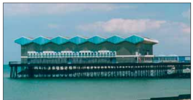
The present sports hall pavilion.
