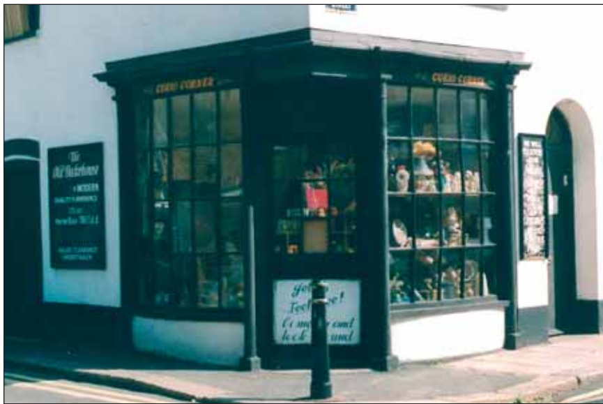
Regency shop front at the corner of Charles Street and Little Charles Street. The chamfered corner for the shop door with overhanging square first floor corner above later became a motif widely repeated through the town.
