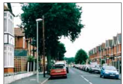
Looking south along Downs Park. Quality townscape.
