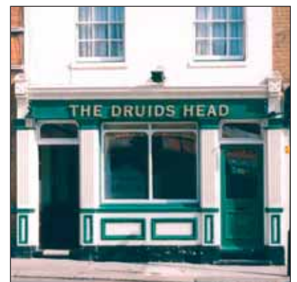
Intact Victorian pub front in Regency house, Bank Street.
