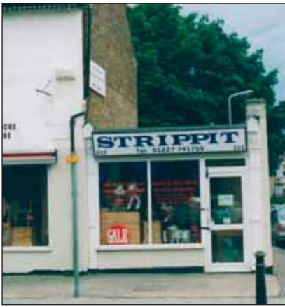
Single storey shop, High Street.
