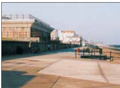
Promenade. View west from sewage pumping point showing key north projecting development block beyond Kings Hall.
