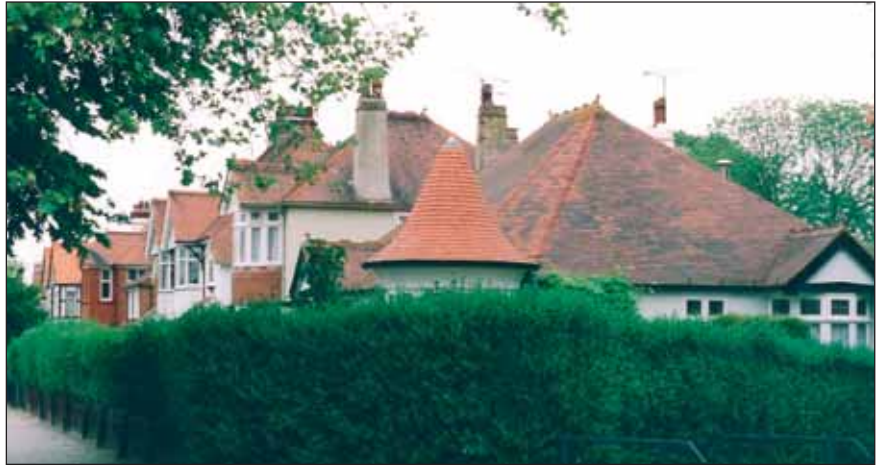
Station Road. looking north. Quite high quality materials and design in this suburban context.
