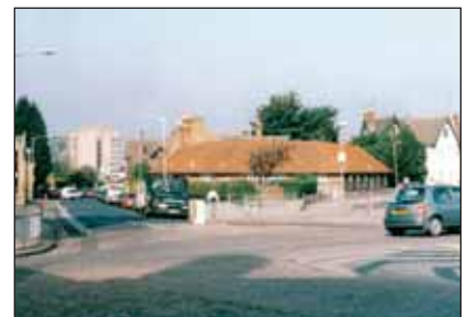
Mickleburgh Hill/Canterbury Road junction, looking west down King Street. Failure of enclosure on north west side.
