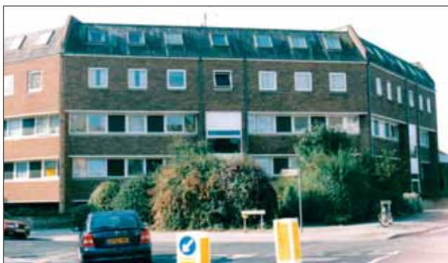
The 1960/70s four and a half storey 'corner turning' flat block on the corner of Station Rd and Western Ave., seen from Western Ave.
