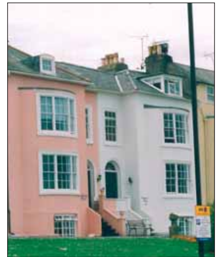
Unaltered pre1840 houses, Marine Terrace
