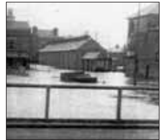
Flooding seen from High Street, 1897 (Gough)
