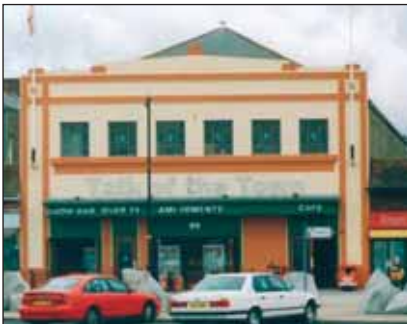
'Talk of the Town', the Promenade, refurbished façade.
