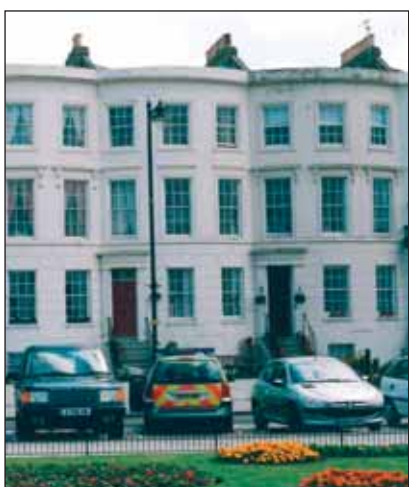
Three bays of Telford terrace on Central Parade.
