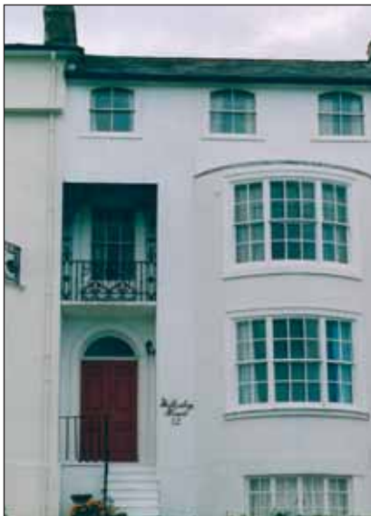
Stuccoed house, 1825, Marine Parade, original detail with added Victorian top floor. Note glazing division differences.
