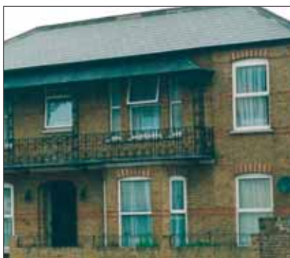
Double bay fronted villa at east end of High Street. Iron balcony has affinities with the Regency style, 1879.
