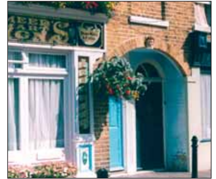
Ornate glass panelled 19th century inserted shop front, Bank Street.
