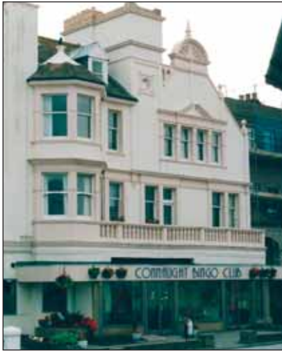
The former Connaught Hotel, Central Parade, 1890s. Originally brick and 'stone dressed' construction with classical arched ground floor.
