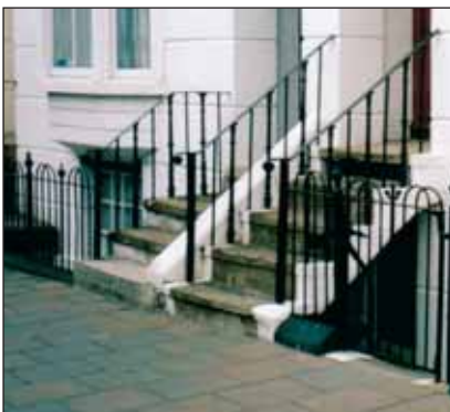
Original 19th century railings, Mortimer Street.
