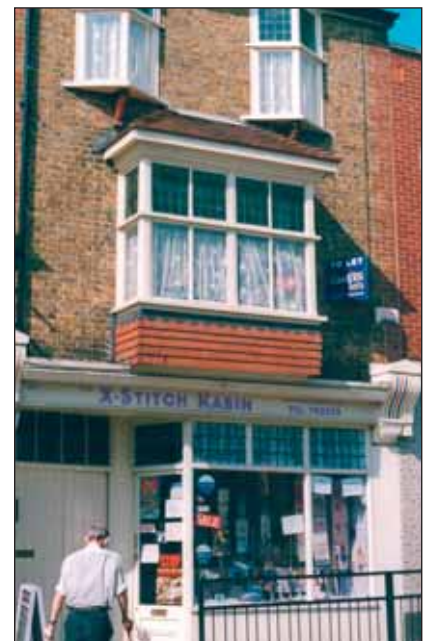
Post Great War. Two high level bays, one at first floor, High Street.
