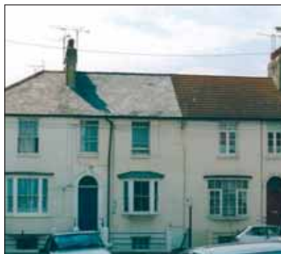
Terrace of 4 in Richmond Street, facing up Mortimer Street, 1863. Original form of cantilevered bay window is on left. Somewhat mutilated.
