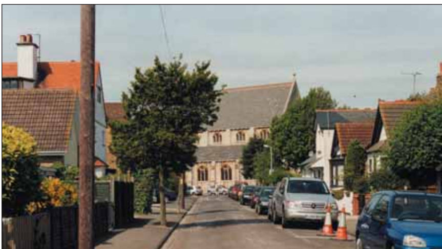
View west along Montague Street to south east flank of Catholic Church. Trees important in streetscape.
