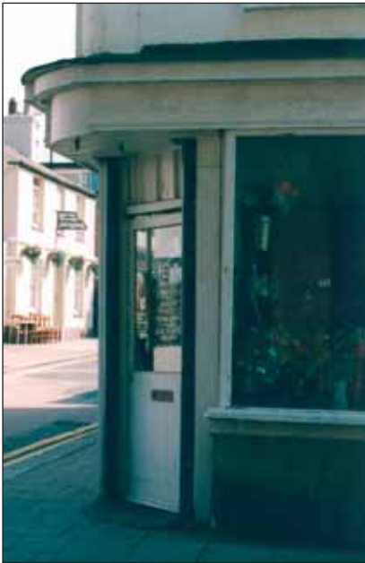
Above: Early chamfered ground floor entrance, rounded corner above, Charles Street/Little Charles Street. Note shallow depth fascia for signboard.
