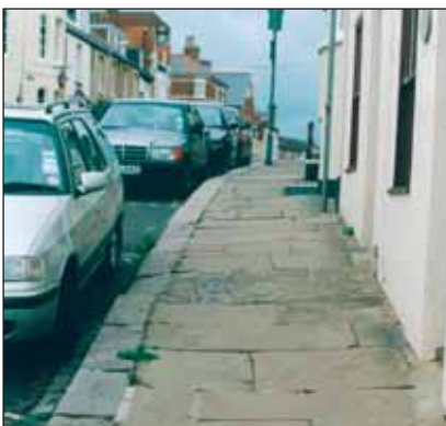
Original York Stone paving and granite kerbs, East Street.
