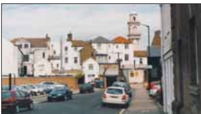
The 'end' of Beach Street – two more town centre car parks with no redeeming features. The surrounding house backs could become genuinely picturesque once more if their originally designed character was reinstated.
