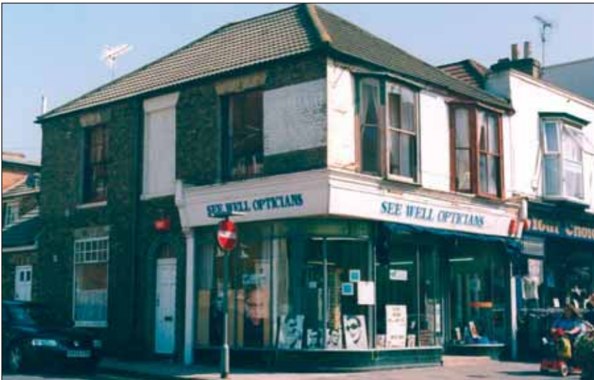
Left: much altered regency house, corner William Street/Charles Street. The corner of the original brick building is held up, within the inserted later shop front, by a series of circular steel columns set behind glass
