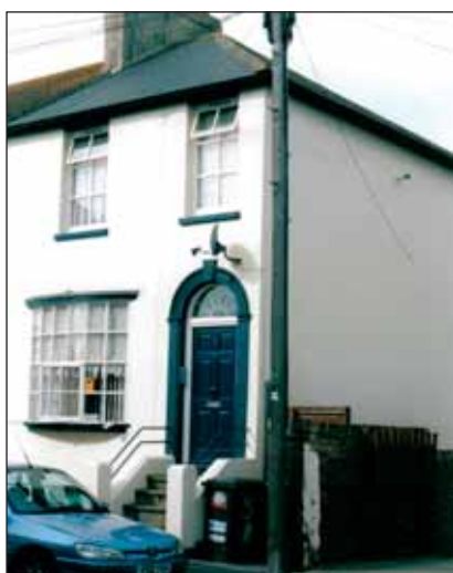
An unlisted house of the 1840s with surviving original porch detail, including door and fanlight, and much damaged windows and area railings.
