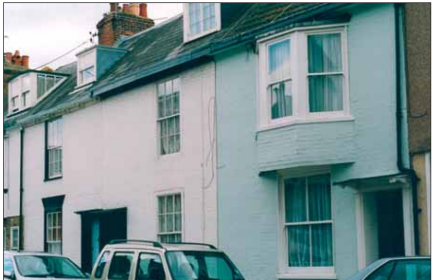
Unaltered 1816 terrace house, East Street. Note surviving dentilled eaves gutter and small dormer.
