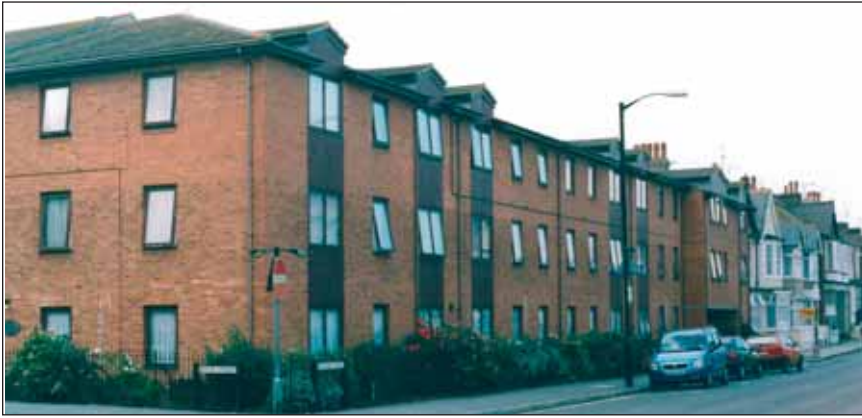
Modern slab sided housing block, Mortimer Street. 'Bays' have become flush strips up the walls and 'gables' have shrunk down and retreated behind the gutter line.
