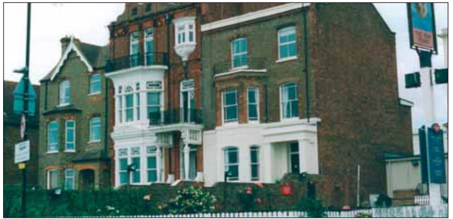
Right: Three storey terrace with ostentatious two storey curved sided bay window and porch (balconies over) and oriel window, 1885. Central Parade.
